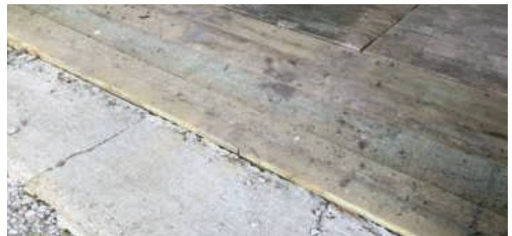
Floorboards were replaced in the entryway
