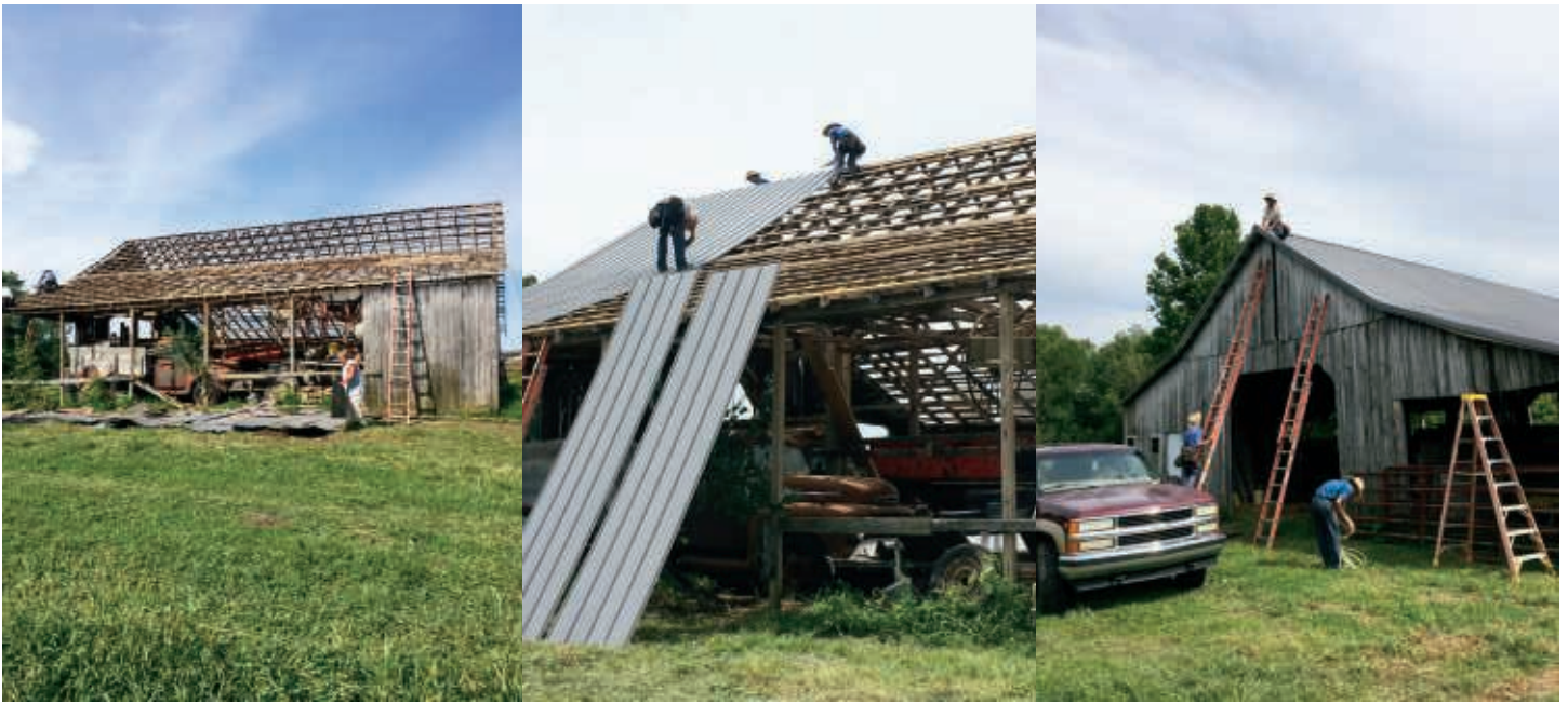
The Amish crew replaced a lot of the boards beneath the tin with poplar boards we had sawed at a local sawmill. They completed the roof in one day. I think it looks great
